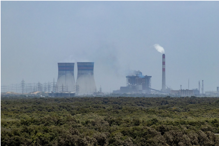
A power plant and industrial site: short-run aggregate supply depends on production costs
