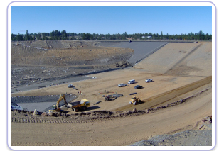
Landfill: line, capture leachate, manage methane
