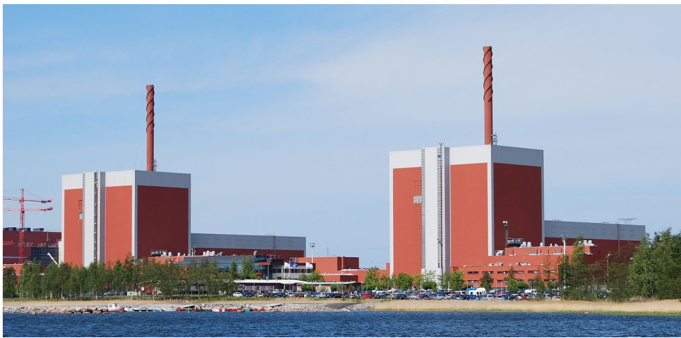
A nuclear power station. The reactor buildings hold the fuel; the sea supplies cooling water. Notice there is no smoke — fission releases no CO 2
