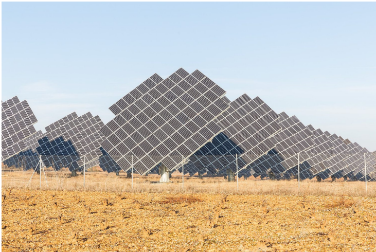
A solar farm. Rows of photovoltaic panels are tilted toward the sun; a big output needs a large area of land
